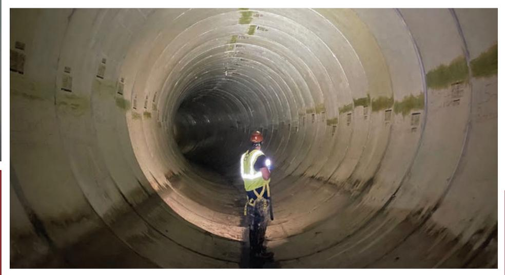
In June 2020, the Pilot Project was put out to bid for 1,560 LF of the PCI-4 Interceptor and Channeline was specified as a mandatory rehabilitation method. Low-bid contractor Marra Services of Cleveland Ohio chose Channeline to supply 1,280 LF of multi-segmental fiberglass liner with the proprietary Tapered Tongue-and-Groove Jointing system.
